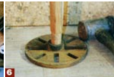
6 Dowel forming the old way
